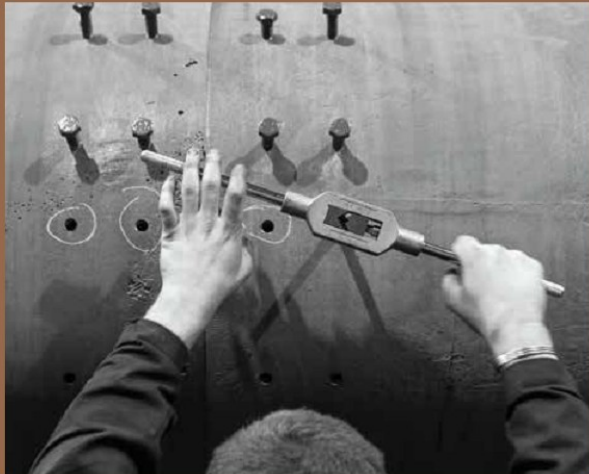
It has taken over two years to painstakingly refurbish the 123 cast-iron gasholders columns
